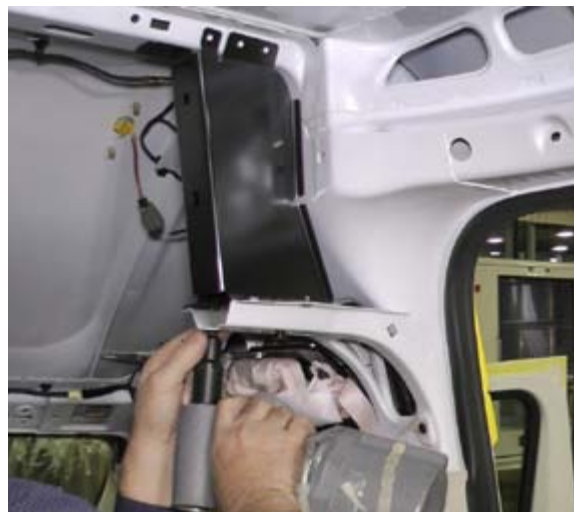
Secure gusset with blind fasteners
