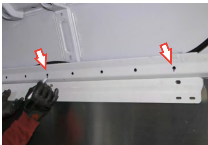
Align sidewall hex holes with rail holes
