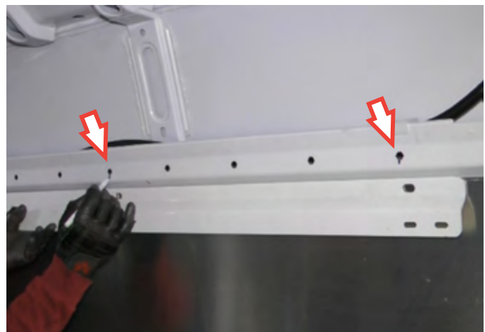
Align sidewall hex holes with rail holes
