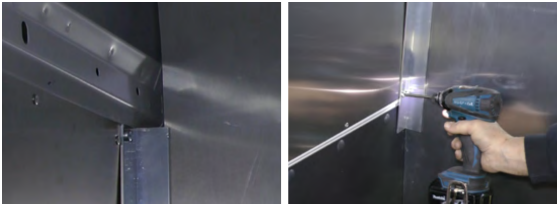
Screws in vertical angle
