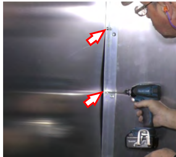
Fasteners in closeout panel and angle bracket
