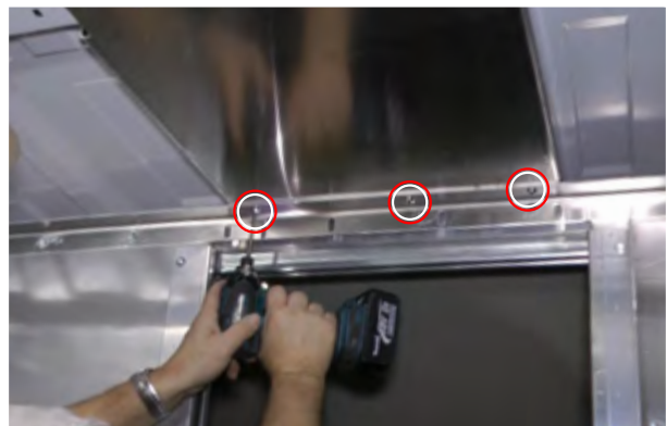
1/4-20 fasteners in roof brace
