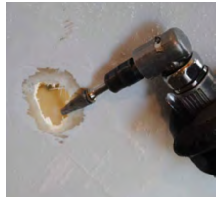
Grind damaged section.
