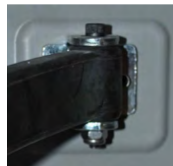
Replacement bolt and nut on strap
