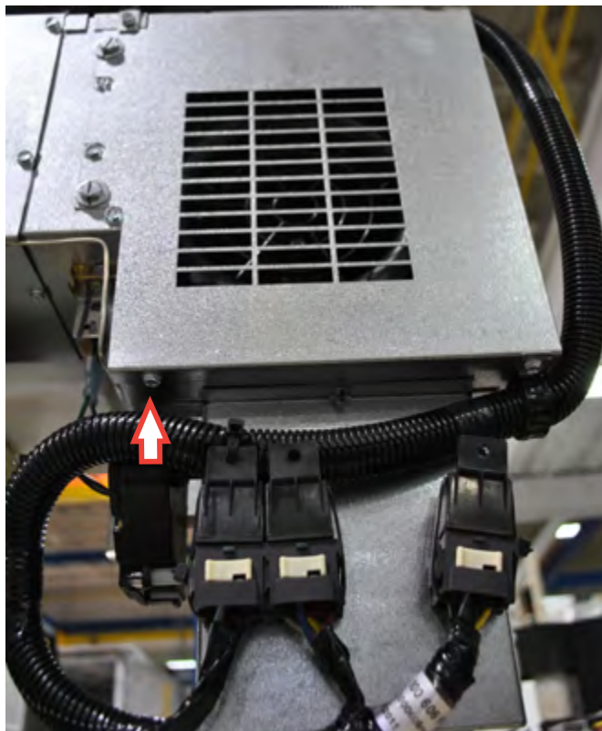
Screw on blower motor housing
