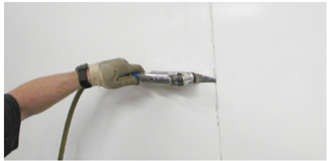
Cutting adhesive in seam with windshield removal tool
