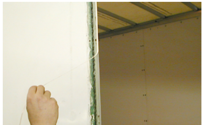
Removing tape backing (exterior seam side)
