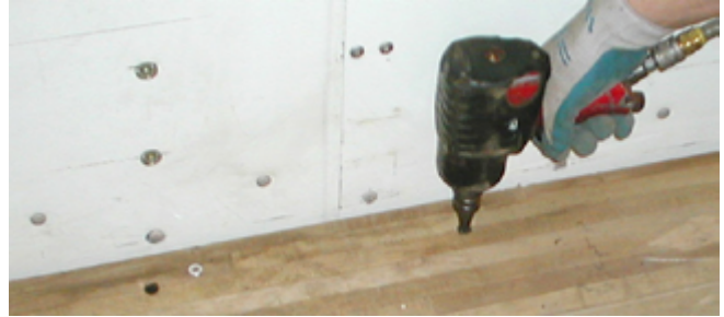
Removing floor plank fasteners
