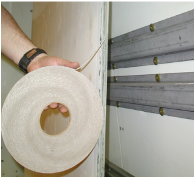
Applying foam tape (interior seam side)
