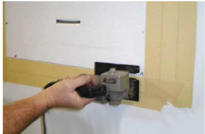
Mark off damaged area and cut out
