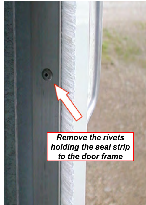
Brush seal on roll-up door
