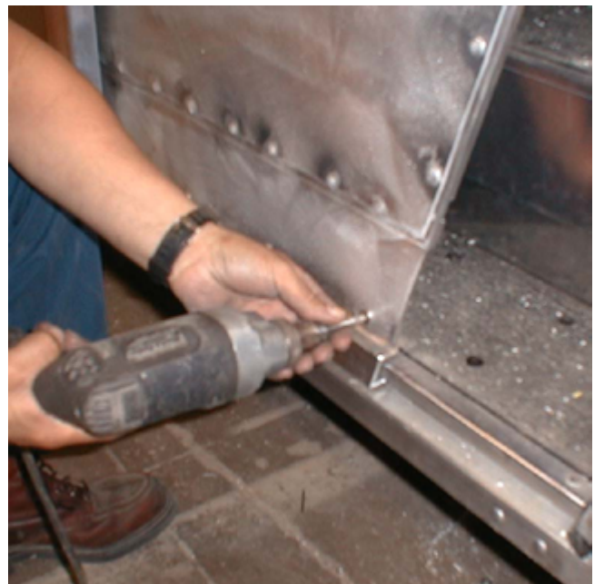
Remove bottom screws
