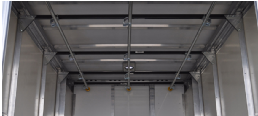
Linen (pipe rack) package
